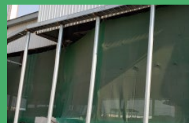
Dust screen has been installed around the lithium slag storage yard
